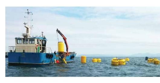
Albatern is a wave energy technology company which develops novel offshore marine devices: buoyant "Squid" modules with three arms that are each capable of linking with up to three other such Squids. The linking of three Squid devices forms a hexagonal arrangement, and these can interlink to form arbitrarily large "Wavenet" installations.
